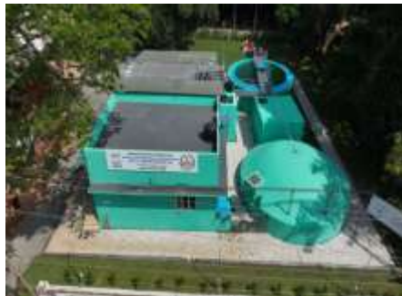
360 KLD STP at General Hospital, Thrissur
